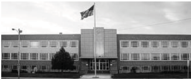
Bannock County Courthouse
